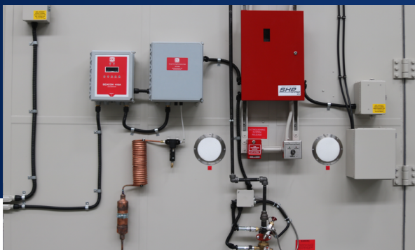
Gas Measuring system for H 2 , O 2 , & CO
