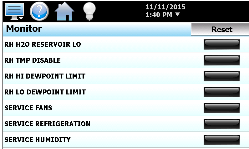
Figure 2-10 System Status Monitor
