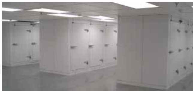
BioStore Freezer Rooms
